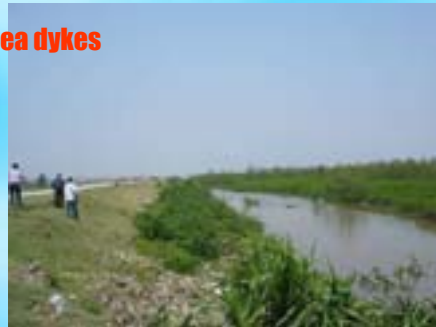
5km of seadyke protected by mangroves in Thai Do Commune and therefore, not eroded in presence of the storm Damrey (Photo: Phan Hong Anh taken on 10/10/2005)
