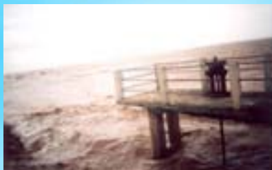
Storm Damrey reaching Hai Phong City
