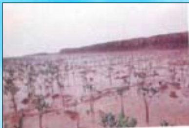
Sea dyke was broken due to the loss of mangrove
