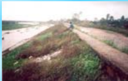
The area behind Bang La Mangroves at 9h30, 31/7/2005, the storm waves can't hit the seadyke
