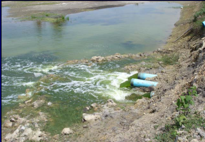
Drain effluent to aeration pond
