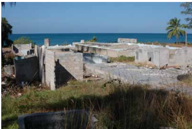
Fig. 8 Shrimp hatcheries were damaged
