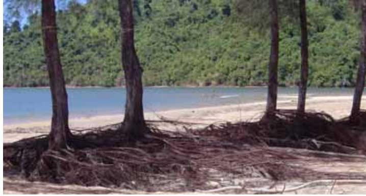
Fig. 29. Trees uprooted as a result of sand erosion (Courtesy of the Department of Marine and Coastal Resources)
