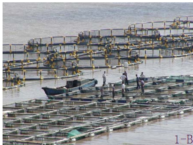
Fig 4 HDPE floating circle cage (1-A, 1-B)
