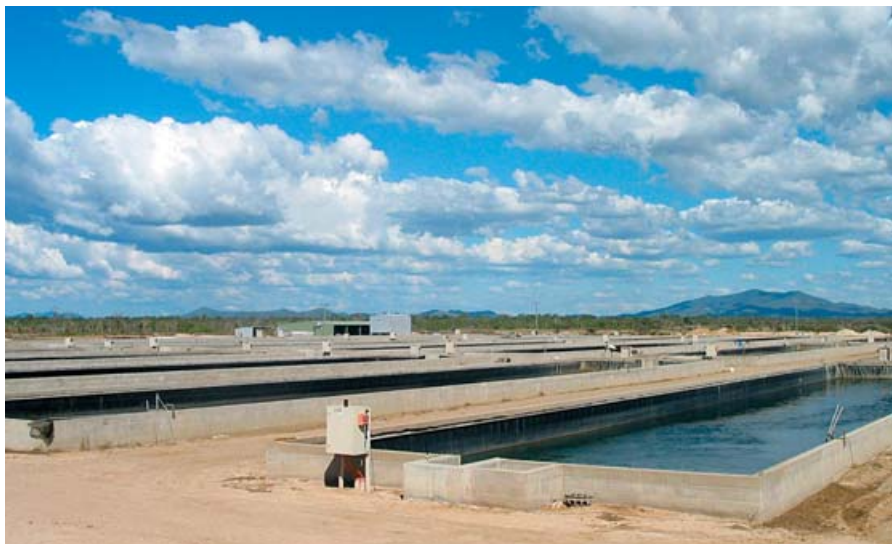
Grow-out raceways at the Good Fortune Bay facilities, Bowen, Australia.
