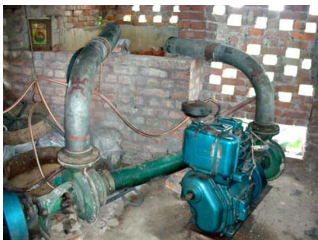
A large farm-level sewage pump.
