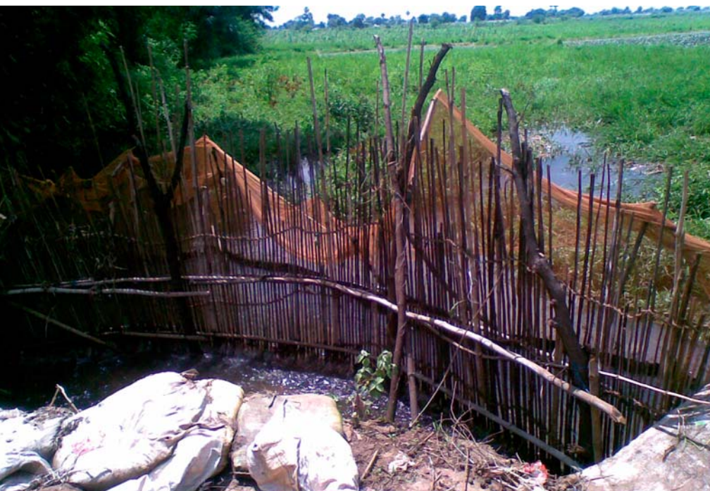
Screens installed to prevent entry of unwanted fishes prior to stocking.
