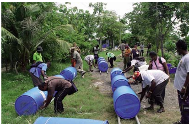
Fixing floats to cage frames.
