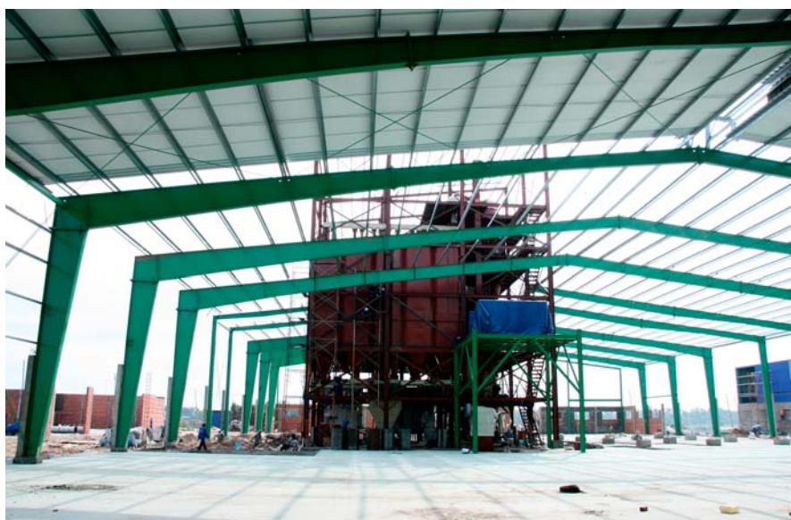
The growth of the catfish industry is fueling expansion of feed manufacturing plants.
