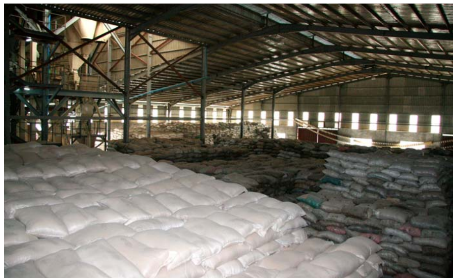
The Htoo Thit Pellet factory - ramping up capacity to 1,000,000 tonnes/year to meet the growing demand for pellet feed.
