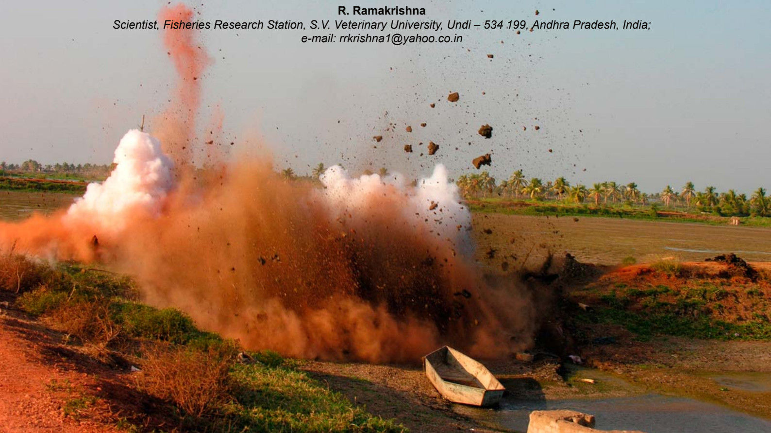
A trial blast to demolish unauthorized fish ponds encroaching a designated wildlife sanctuary.
