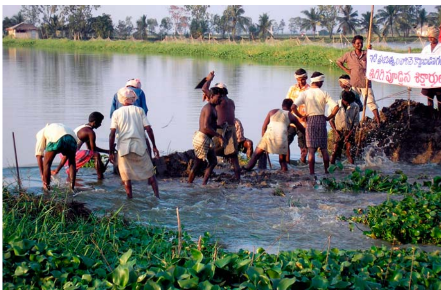
Manual breaching of fishpond embankment, (a warning banner can also seen).
