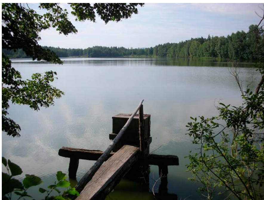
A traditional wooden drainage monk on a fish pond, Czech Republic.
