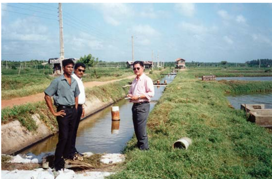
(3) Waste water channels are planted with seagrass for bioremediation of nutrients
