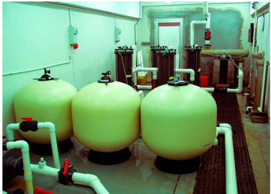
Seawater treatment system for live food.
