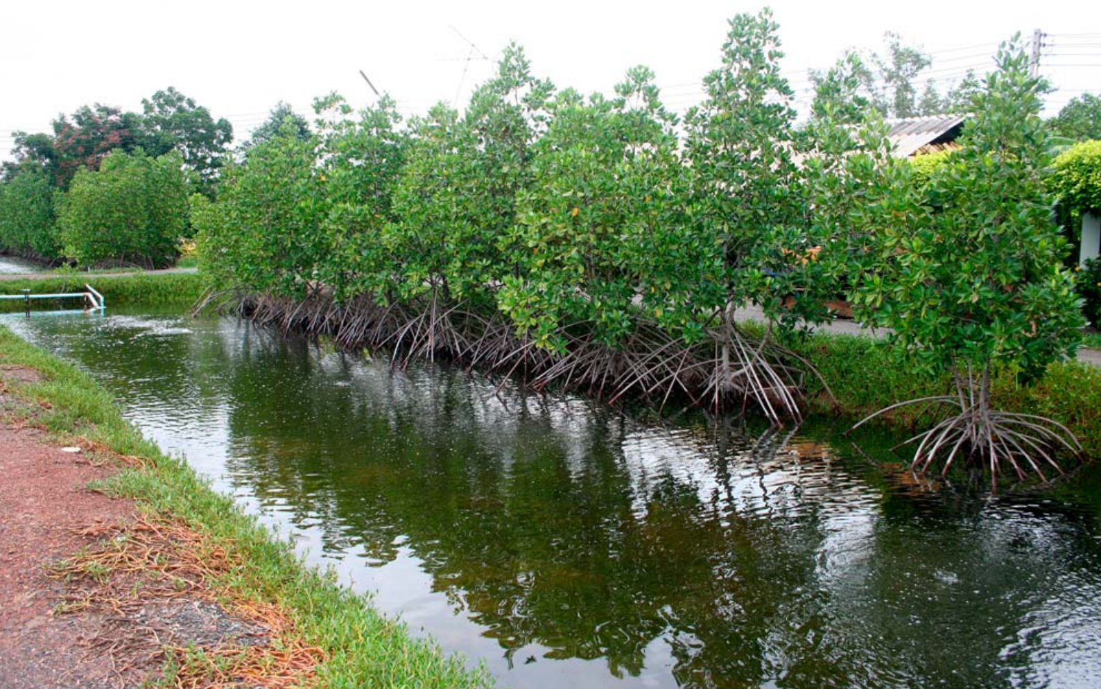
Water treatment canals and ponds are aerated and lined with mangroves to assist in improving water quality. The dykes are lined with 'pigface', a hardy and salt-tolerant plant, to reduce erosion.
