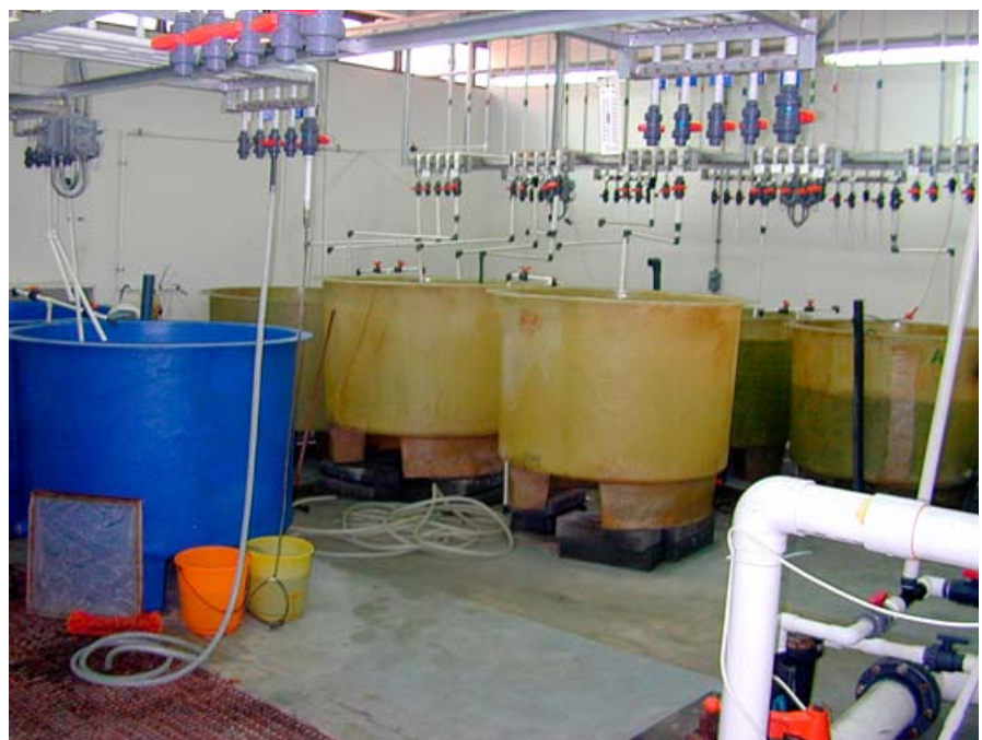
Rotifer chemostat production facility.
