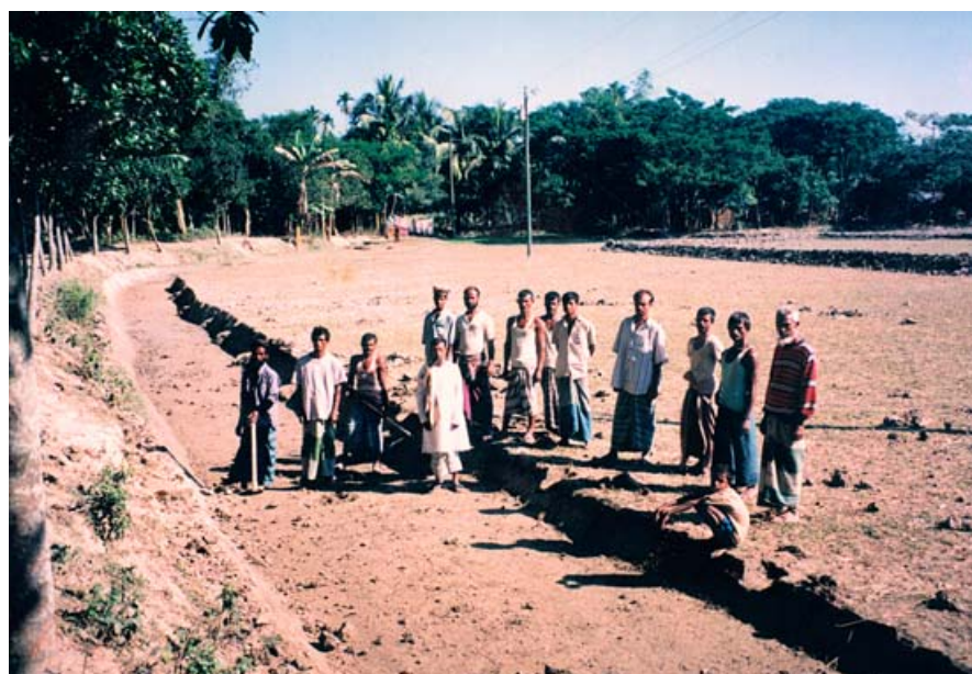
A large dyke for community rice-fish activity being built by a group of farmers.
