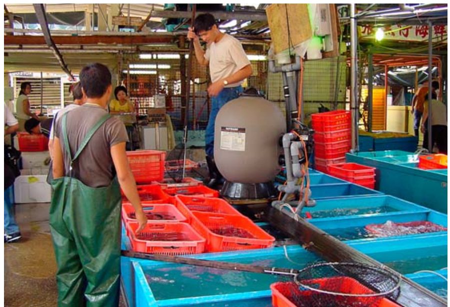
Live fish stall at Aberdeen market using sandfilter to keep the water at the holding facility in good condition.
