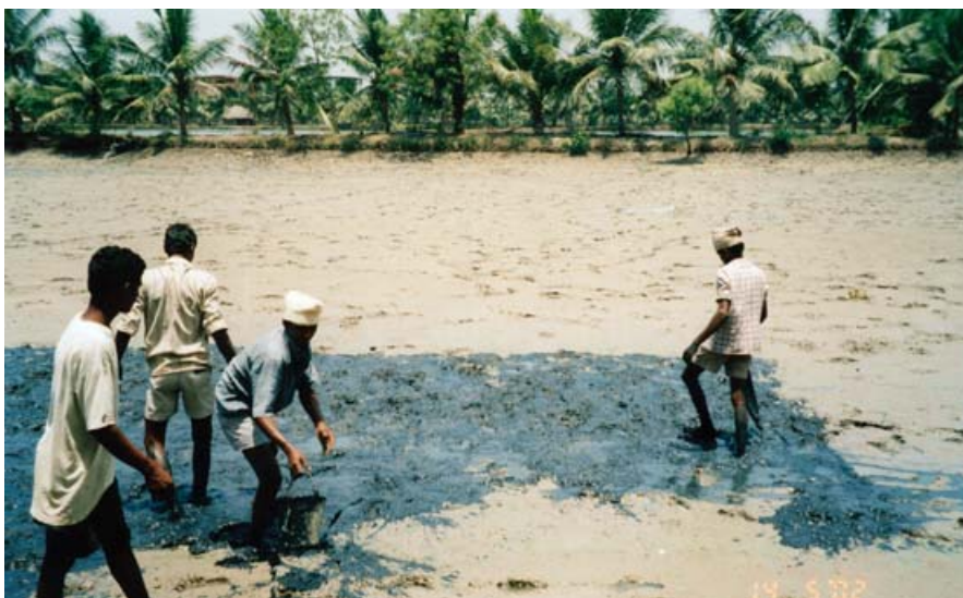
Manual removal of sludge
