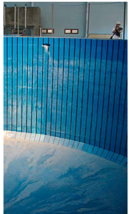
The tuna tanks are deeply inset into the ground
