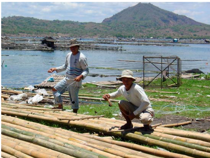
Constructing a cage frame with bamboo.
