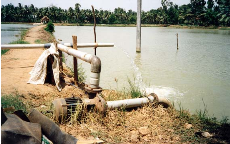
Water evaporation and seepage loss is maintained by pumping ground water in many cases.
