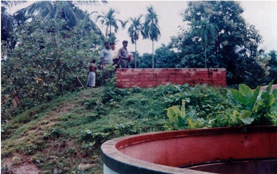
Figure 2: Low-cost overhead tanks are built on piles of earth excavated during pond construction
