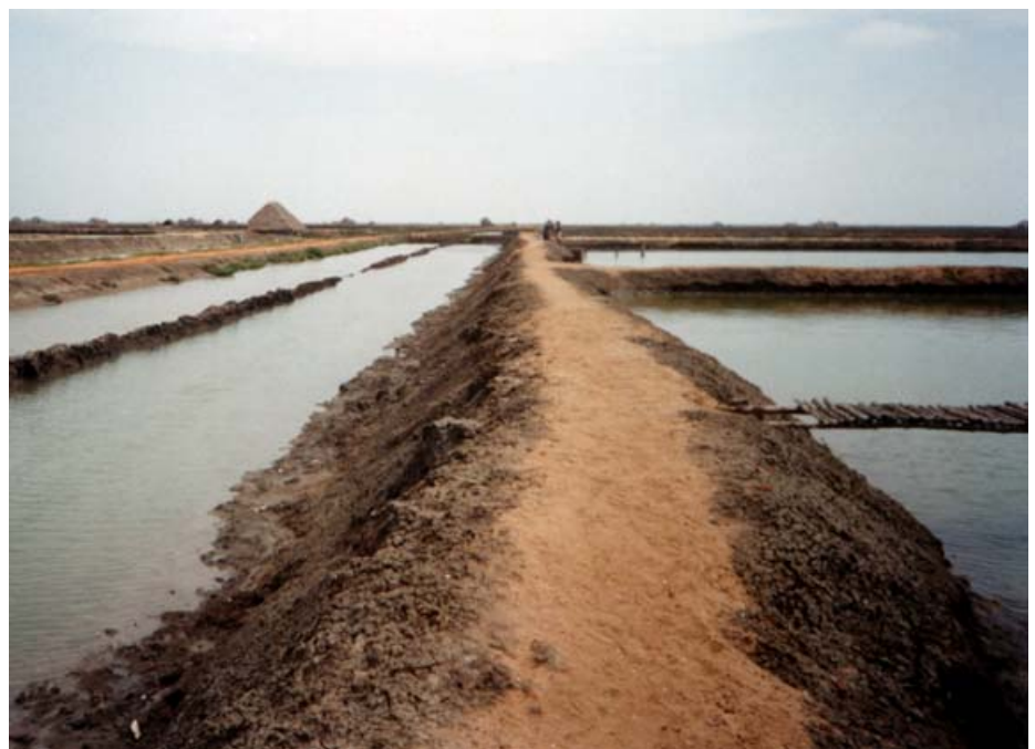
Common infrastructure - inlet canal
